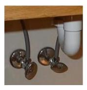
Once a year, fully operate the valves to the closed and opened position once or twice. When you are done, fully open it once more before closing it down a ¼ turn. Moving these valves sometimes releases loose sand or minerals into the water line to a faucet, so remove and clean a faucet aerator as well.
