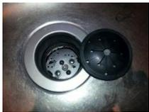
If you have a removable drain baffle, remove it and clean the surface thoroughly with an old toothbrush, water, and detergent. Be sure to place the baffle back into its original location prior to operating the garbage disposal.
